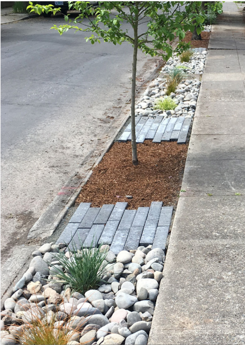
FIGURE 9.2 - STRUCTURAL BMP - EXISTING CURB YARD REVISED TO COLLECT STORMWATER FROM THE STREET
