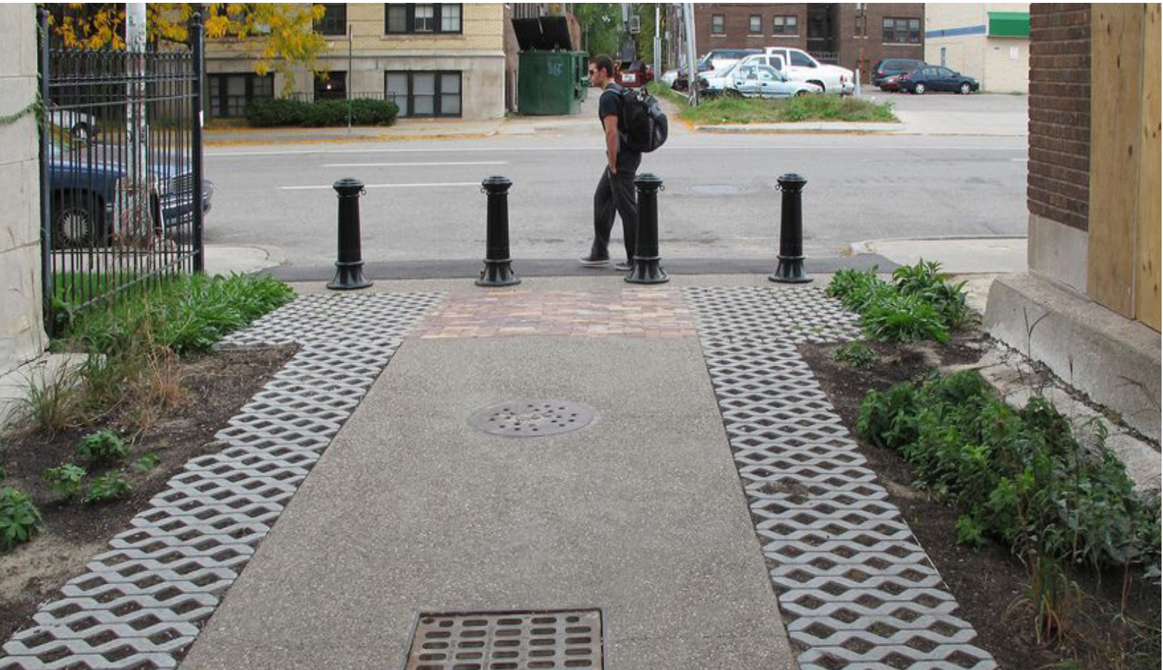
FIGURE 9.5 - EXAMPLE OF A GREEN ALLEY CONVERSION SHOWING BOTH REDUCED PAVEMENT AREAS AND POROUS PAVEMENT
