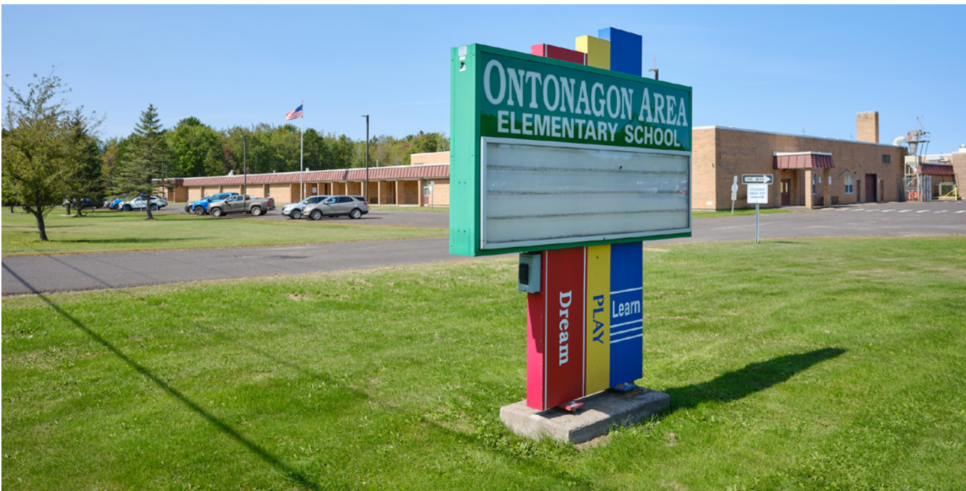
FIGURE 5.2 - ONTONAGON ELEMENTARY SCHOOL
